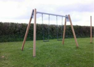
The chain openings are in excess of the 8.6mm as recommended by BS EN 1176 Finding:
