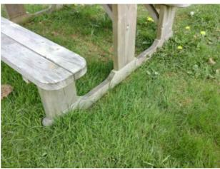
The bench is not securely fixed to the surface **Action:** and there is some possibility of the item tipping or rolling over Finding:
