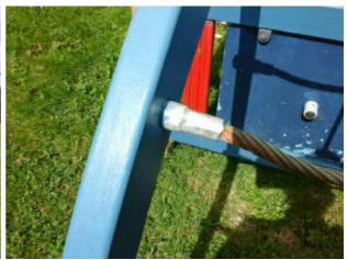
Finding: A number of rope fixing(s) have worked loose **Action**: Secure all loose fixings
