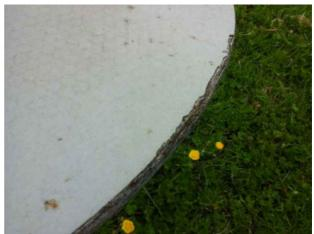
**Finding:** Parts of the timber are rough or splintered
