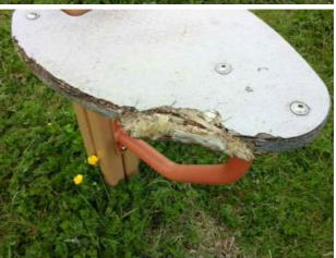
**Finding:** There are areas or parts of the timber stilt platforms on the structure that have rotted around fixing points
