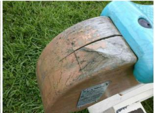
Finding: The plywood has delaminated in some places Action: Remove all rough or splintered edges.
