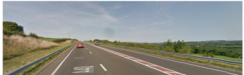
The photo above shows an example of the future layout of the NDLR WS 2+1.
